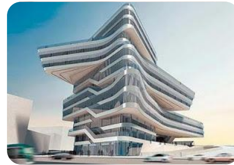
Figure 43 Torre Espiral, Barcelona
