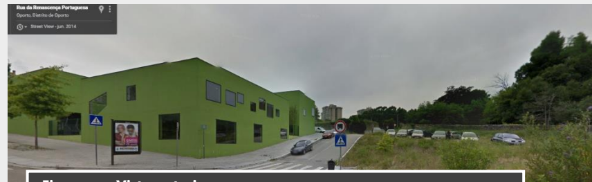
Figura 157. Vista exterior Fuente: Recuperada de https://www.google.com/maps/@41.1652244,-8.5862079,3a,75y,3.27h,88.27t/data=!3m1!1e1!3m1!1s2Kl3cRBa7kM_msVcO!1s2Kl3cRBa7kM_msVcO
